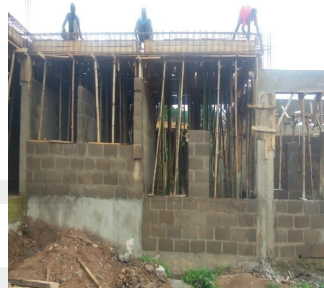
PLATE 1: STAGES OF CONSTRUCTION AT SITE A
