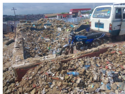
PLATE 3: WASTES FROM DEMOLISHED STRUCTURES
